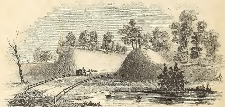
FIG. 20.—VIEW OF GRADED WAY NEAR PIKETON, OHIO.
